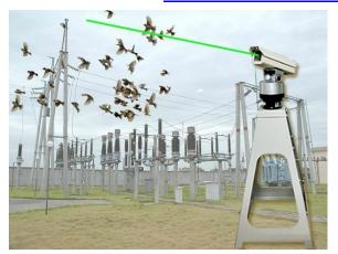
Fig. 4 Laser Bird deterrent
